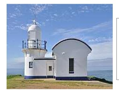
Location: Port Macquarie NSW <u>Coordinates</u>: <u>31.4755°S 152.9372°E</u> Tower Constructed: 1879 Height: 8 m (26 ft) Light Focal height: 34 m (111 ft) Intensity: 12,800 cd Range: 16 nm (30 km; 18 mi) Characteristic: FI (4) W 20s.
